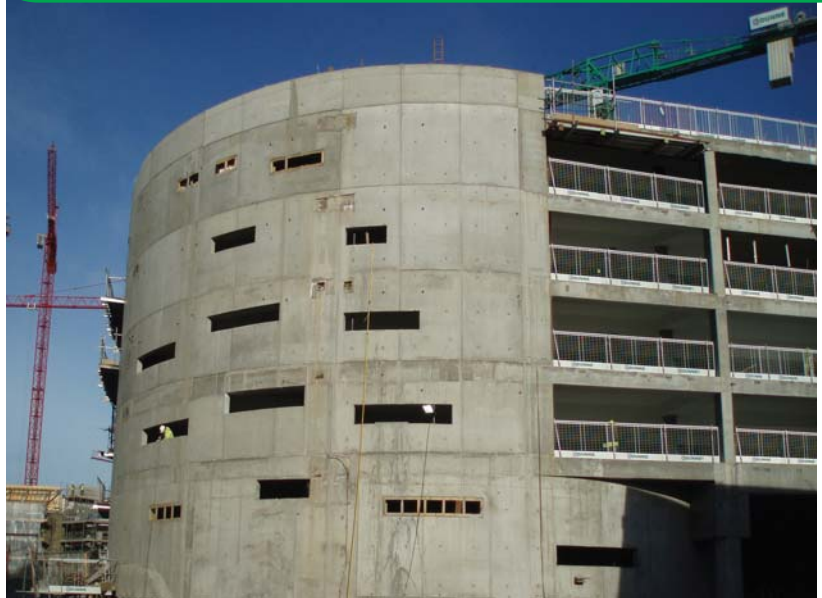
MSCP External view of Rotunda, Paradise Street, Liverpool
