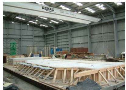
The breaking out of the moulds begins
