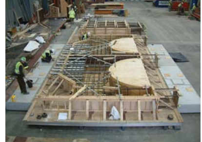
The fabrication of the moulds are completed
